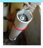
Fill each pipe until it is about 6 or 7 inches from the top - check depth with eye bolt.
