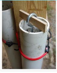
Slide the piece of scrapwood through the eyebolt, then rest it on the rim of the pipe. This holds the eyebolt in place, and prevents it from sinking into the wet cement. (Alternatively, you can fill the cement all the way to the top, then let it set up for a few minutes, then shove the eyebolt into place. I prefer this method as it eliminates guess work and reduces the risk of waiting too long and having the cement set up too long before adding the eye bolt.)
