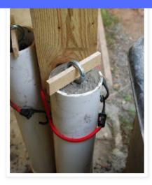
Fill the rest of the pipe with wet cement up to the base of the eyebolt.
