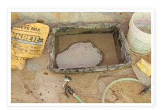
Begin mixing concrete. While wearing a dust mask, dump some of the dry concrete mix into your bucket or tray, then add water slowly. I mixed about 1/3 of the bag at a time, though this depends on what you are mixing in.
