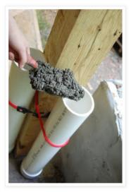
Once a good consistency has been reached, start spooning the mixture into your pipes. (This goes much faster than it sounds!) Every so often, shake or tap the pipe to help the wet cement settle into place.
